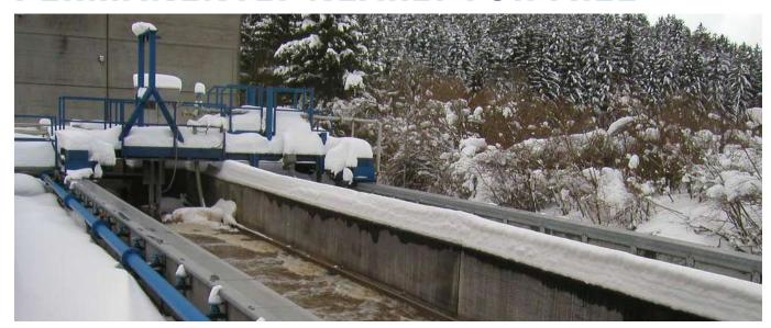
Clearly, a heated scraper runway simplifies the winter operation considerably. What is new about this is that the operating costs of such a heating system are next to nothing because one can dispense with external energy sources. Both pictures show this type of installation; last winter we undertook several extensive tests and the product proved itself superbly. Innovative technology from Krumme GmbH! We will gladly inform you about our products!
