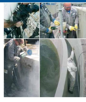
issued by Deutscher Beton- und Bautechnik-Verein e.V. (German concrete and construction association). The experience we have made for many years with all sorts of concrete is supported by machinery operating with the most advanced technology. The 2500 bar water jet apparatus is followed by special concrete spraying machines and coating procedures which form a concrete surface that stands up to close examination.
